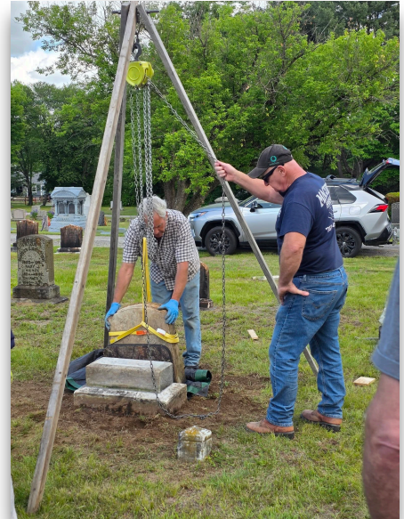
Jonathan demonstrated how to raise and re-set multiple piece monuments using a tripod for heavy lifting.
