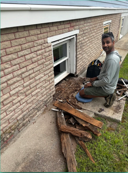
We thank Kumar with Phoenix Builders for replacing rotted window sills at Heritage Hall.
